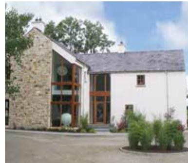
Working closely with architect - Andrew Coulter, Keystone engineer - Chris Patterson, detailed the unique two storey glazed gable apex with a cantilevered balcony, two story corner lintels and half apex corner lintels.
